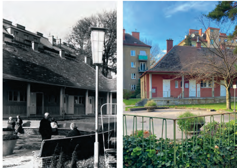
Fig. 6: Heritage-listed Alte-Leute-Siedlung in Steinitzhof (1130 Wien) with a deteriorated central open space that reflects lost communal life—yet holds untapped potential for revitalisation
